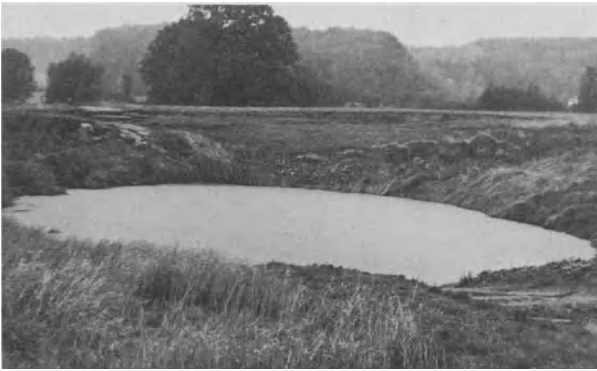
Fig. 22. Subsidence funnel over a potash working collapsed by water penetration
