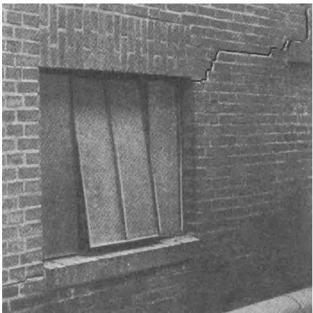
Fig. 5. Gap created between gables (left) in a terrace of houses by convex ground curvature Fig. 6. Shear cracks from mining subsidence which is affecting a partition wall
