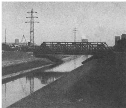
Figs. 1 and 2. Before and after raising a bridge and embankments at a canal where the ground had subsided while the water level remained the same
