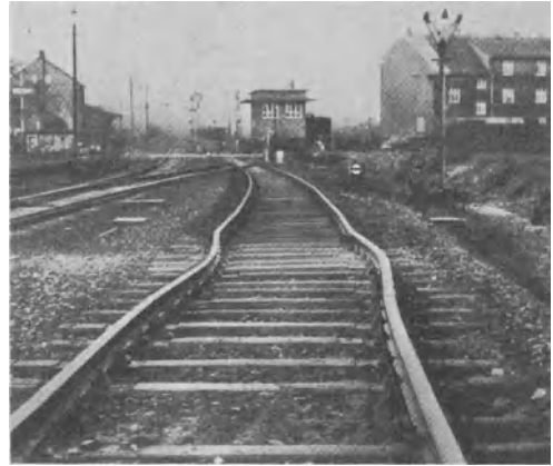
Figs. 10 and 11. Damage to railway tracks caused by ground compression: vertical distortion ( left ) and lateral distortion ( right )
