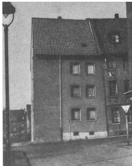
Figs. 3 and 4. Before and after rebuilding the end house of a terrace damaged by concave curvature in a subsidence trough. (Note manner of correcting for tilt at join with next house)
