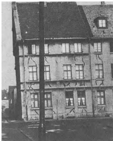
Figs. 3 and 4. Before and after rebuilding the end house of a terrace damaged by concave curvature in a subsidence trough. (Note manner of correcting for tilt at join with next house)
